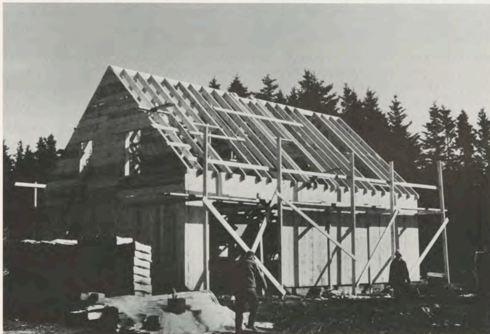
Uses of the timber harvest: dimension lumber for on-island post-and-beam construction.
