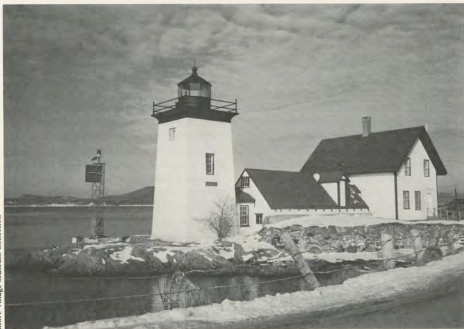
Grindle Point Light Station today. Though the lantern is neither much bigger nor much higher than its predecessor, this tower is more "correct." This is one of the Egyptian towers, with references to Masonic precedents. The picture also shows the present state of the art in lighthouse design.
