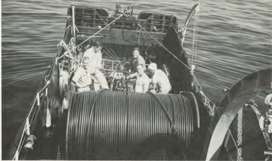
Johansen and his crew aboard the Coast Guard cablelayer.
