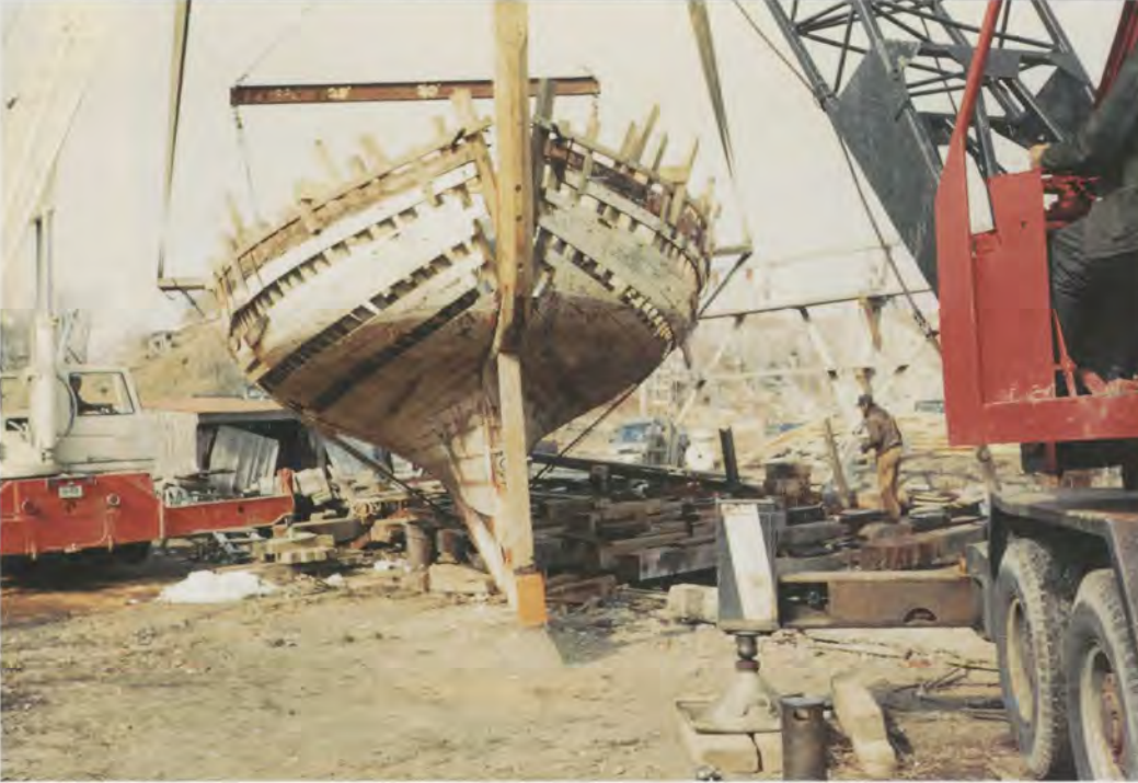
During the rebuild in Rockland, 1991
