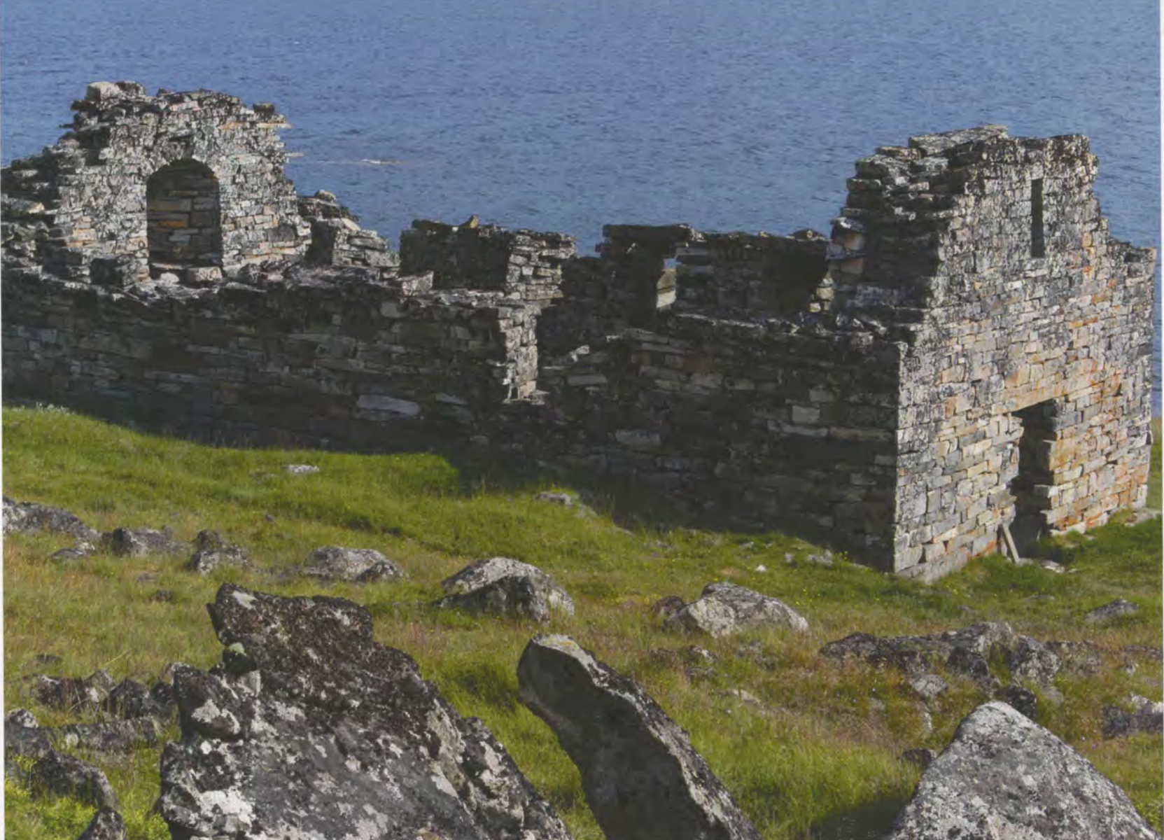
Ruins of the stone church at Hvalsey
